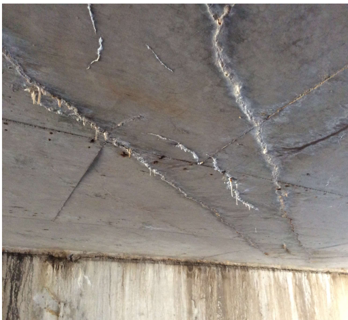
PHOTO 4 Description Typical soffit cracks with efflorescence and staining.
