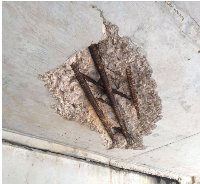
PHOTO 1 Description Span #2 soffit between piles # 5,6.
